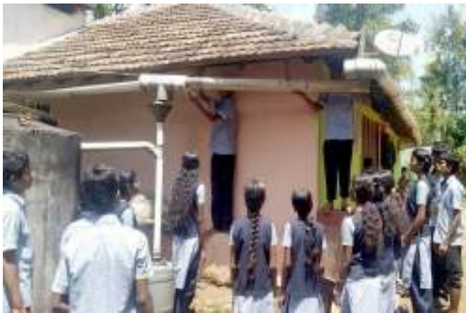
Students install rainwater harvesting structures in Gendethur Village
