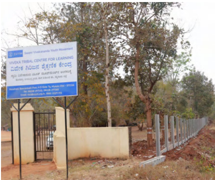
Construction of a Compound Wall to Enhance Campus Safety
