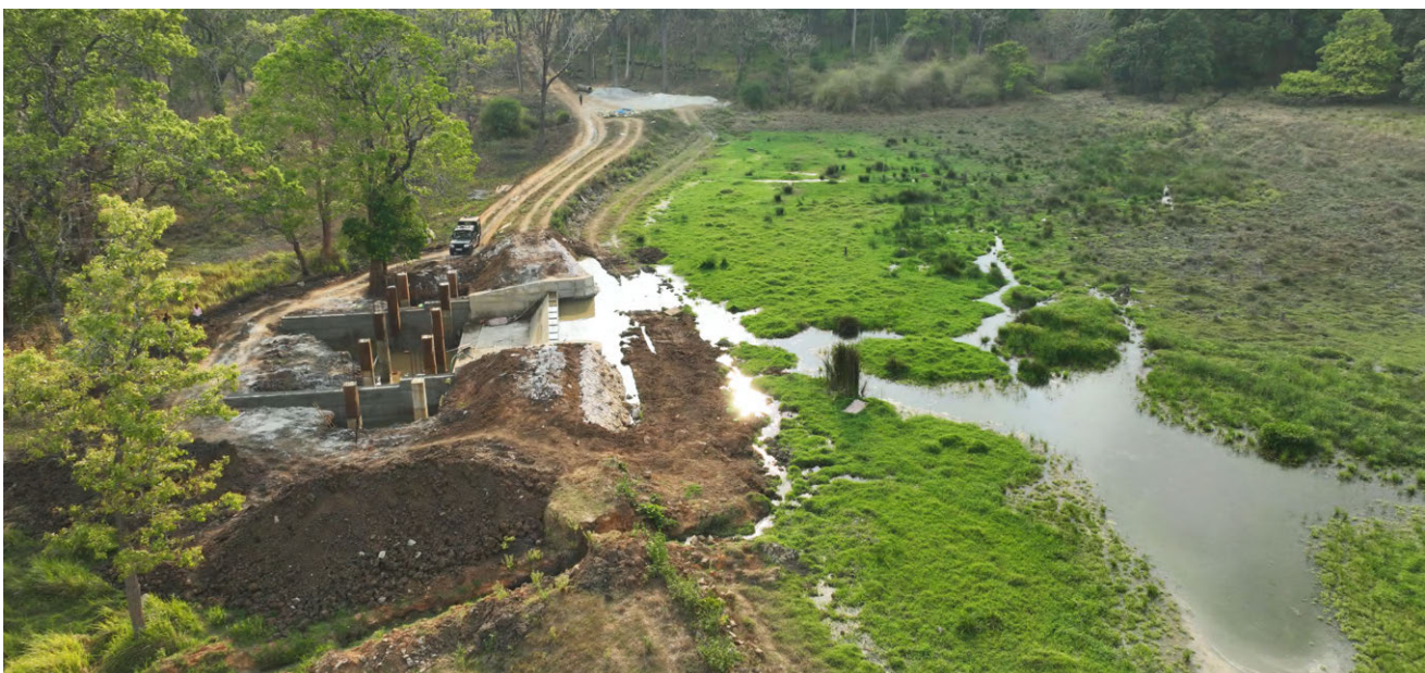
Bridge construction along the Nagarhole Safari Road to ensure year-round access for forest department vigilance, particularly during the monsoon, alongside the construction of a waste weir at Doddhalla Lake to support drinking water availability for wildlife.
